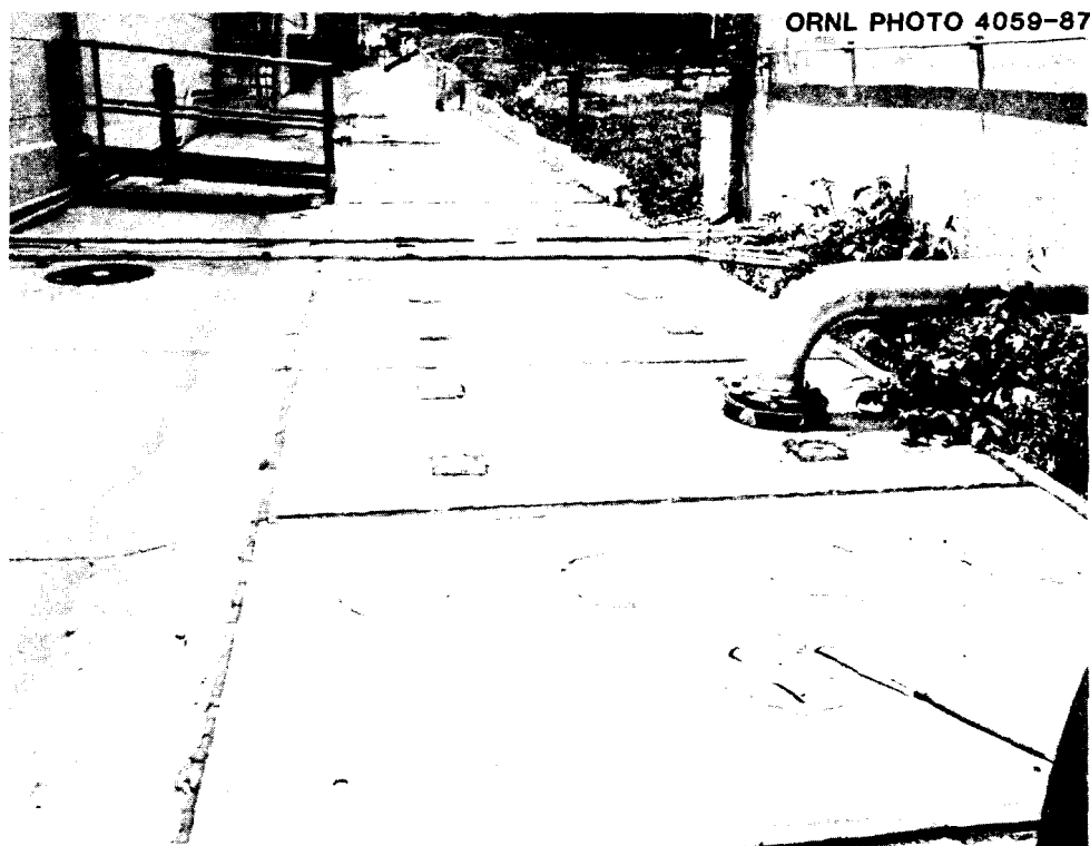
FIGURE 7 DETERIORATION OF CONCRETE VENTILATION DUCT
