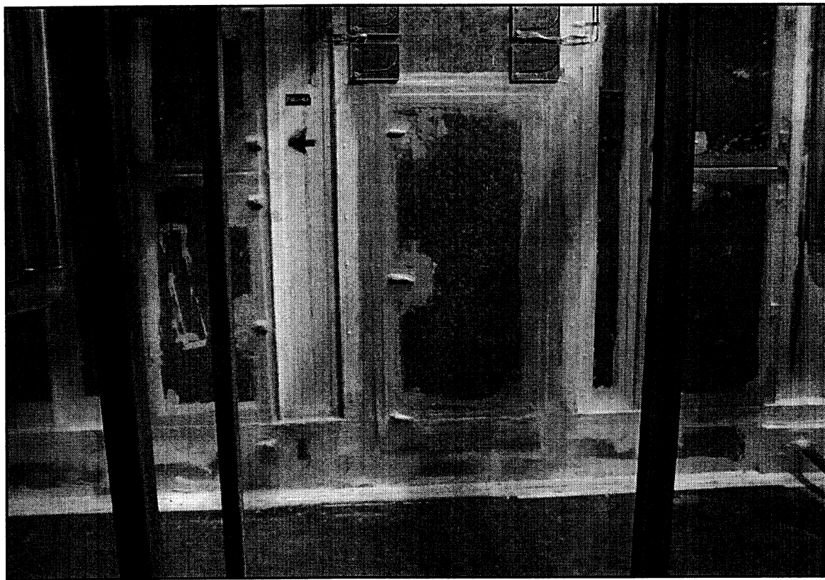
Figure 6 Air Handling Unit access door showing sealant work.
