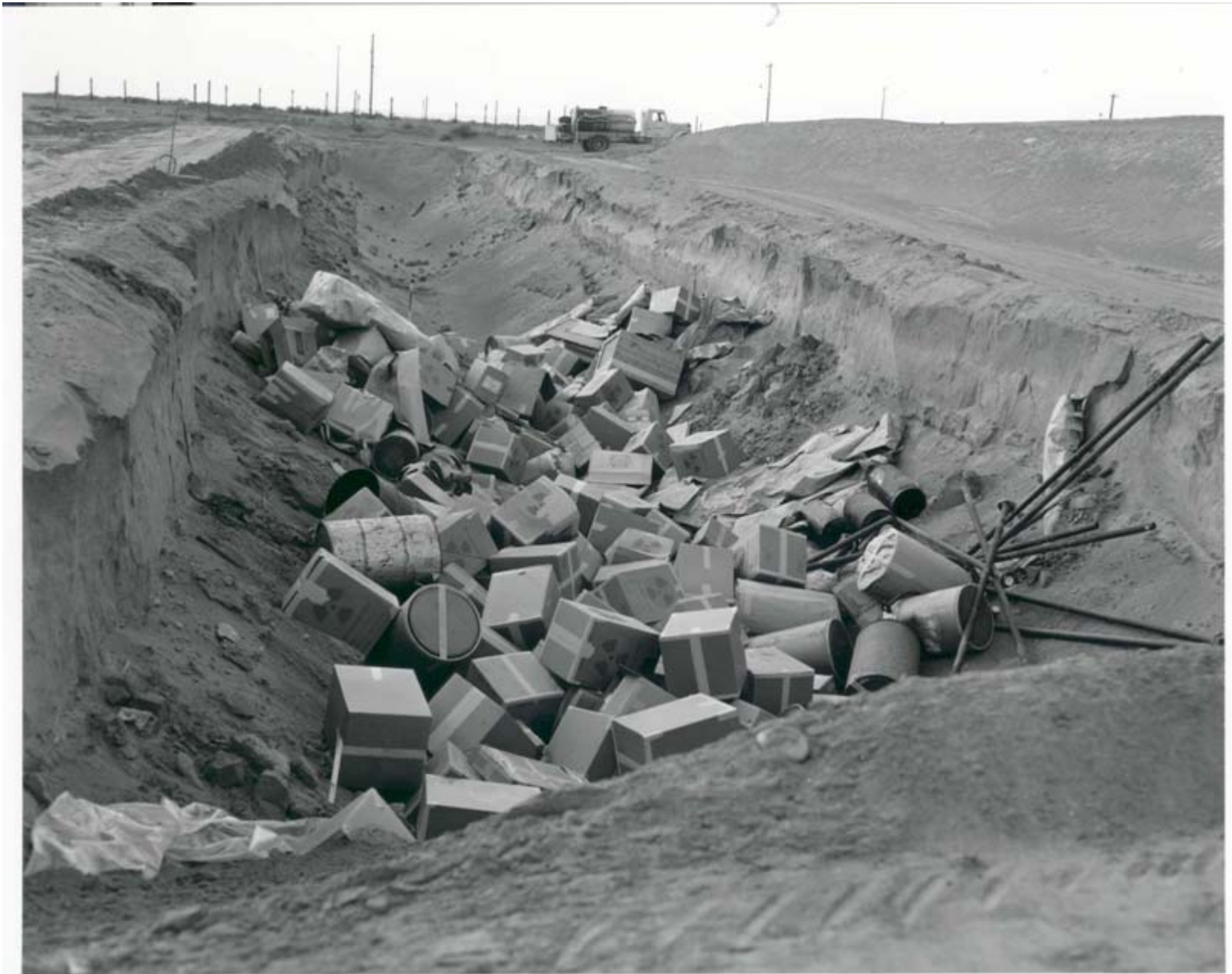
Solid Waste Trench, Hanford, 1953
