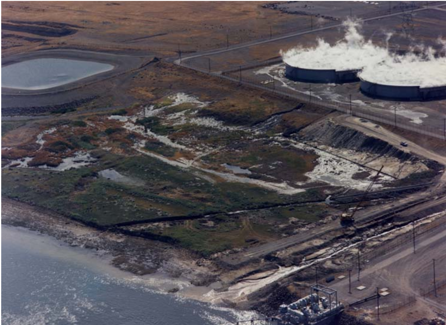
K East Reactor basins overflowing, leaking, 1962
