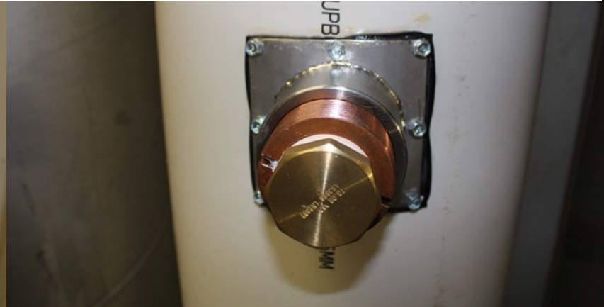
Injection point. Tech Screws in plastic ducts
